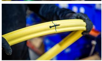
6. INSERT CABLE TIE, TIGHTEN THEN SNIP OFF END **OR** GLUE ENDS USING A STRONG ADHESIVE.
